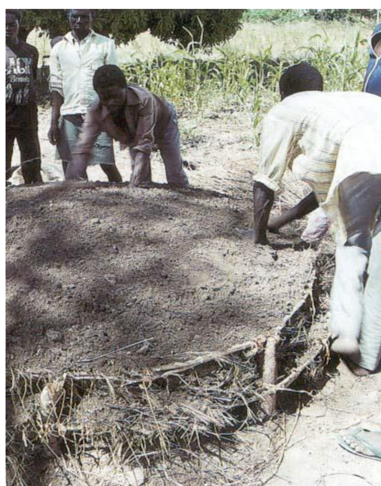
CONSTRUCTION OF THE CLAMP
